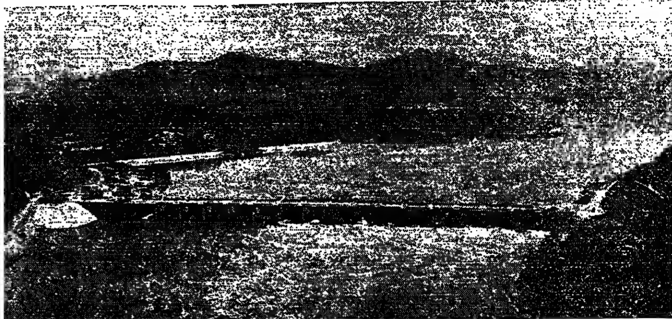
As part of full-fledged government endeavours to explore energy sources a new hydro-power station was built in the northern outskirts of Seoul. The Paitang Dam, featuring the "low-head valve-type" power plant, is the fourth hydro electric plant erected along the Han River.
